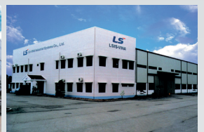
Hanoi factory (Vietnam) MV/LV Switchgear, Mold TR
